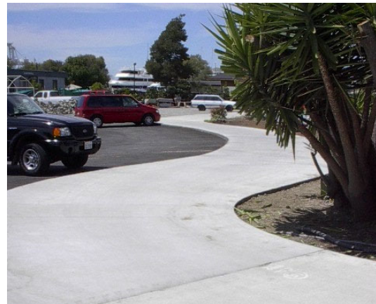
Bike path at Barnhill Marina – 12 feet wide, concrete, circuitous path of travel
