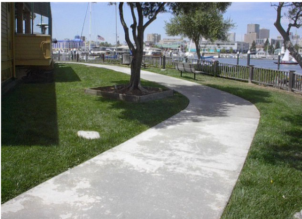
Path east of Mariner Square Dr. – 6 feet wide, concrete
