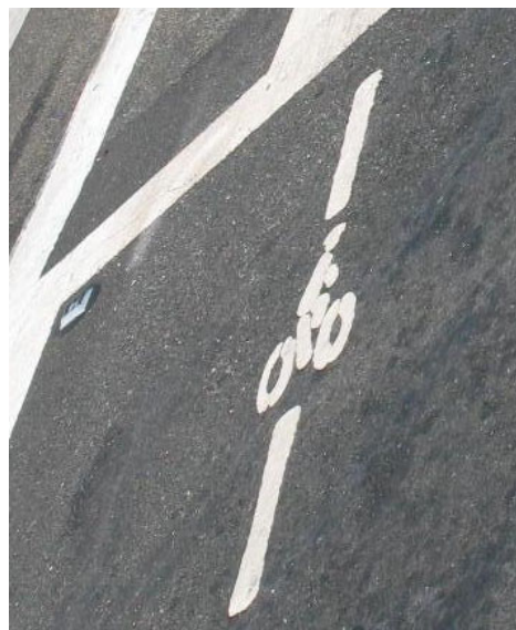
Stencil indicating the proper positioning of a bicycle to activate loop detector at a traffic signal.
