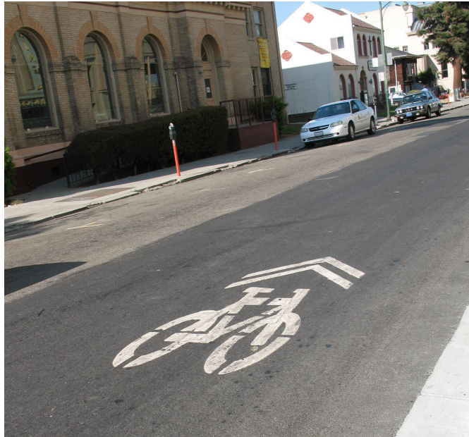
Shared lane marking on Oak Street
