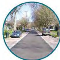
Permeable Pavers in Parking Lanes
