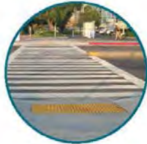
High-Visibility Ladder Crosswalks
