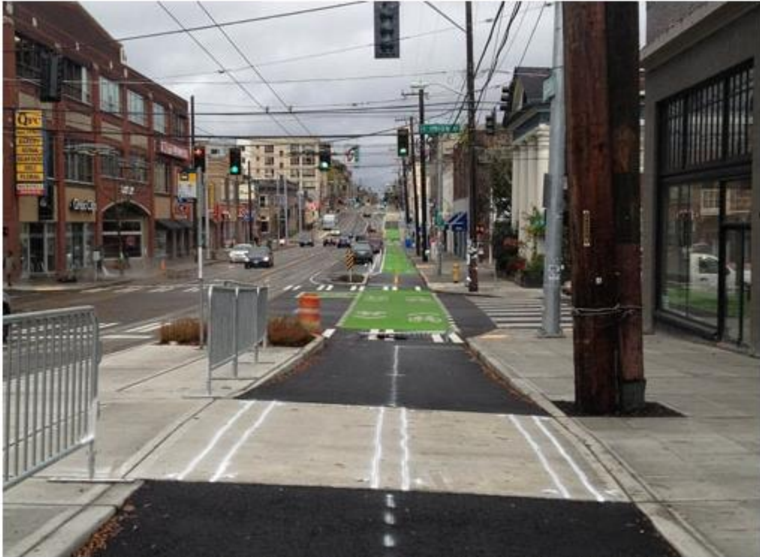
Raised crosswalk (under construction) adjacent to a transit stop island platform on Broadway in Seattle, WA. (Source: Seattle DOT)
