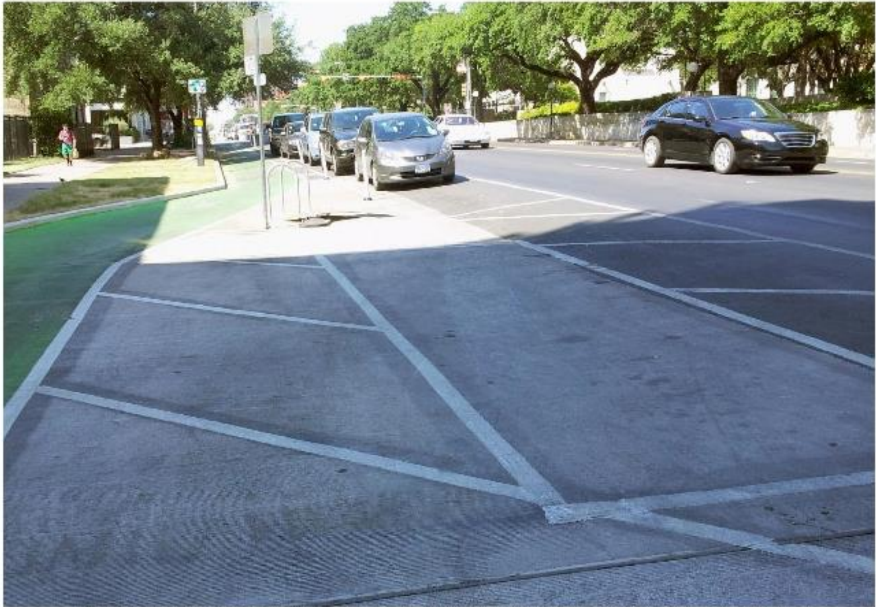
A dedicated accessible parking space with access aisle in Austin, TX. (Source: Kelly Blume)
