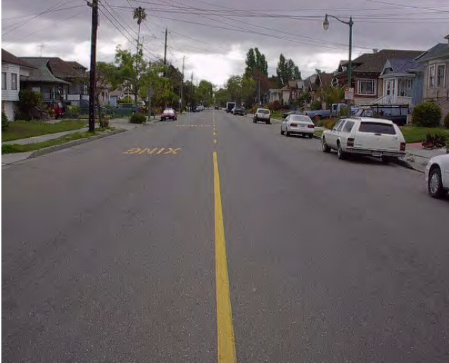
FIGURE V-19. Buena Vista Avenue looking east (Section 5).
