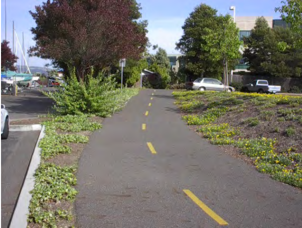
Path connecting Wind River to parking lot at Encinal Yacht Club (north of Trail Section 3, Sheet 6).
