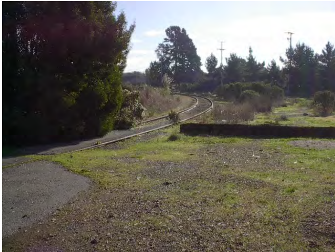
FIGURE V-8. Looking south from Atlantic/Constitution intersection into former Alameda Belt Line Rail Yard (Section 3).
