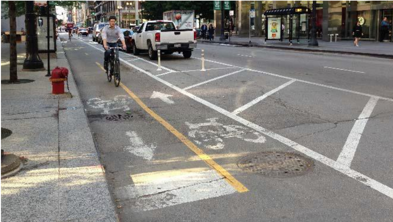
Figure 2: Two-Way Cycle Track on Dearborn Street in Chicago, IL
