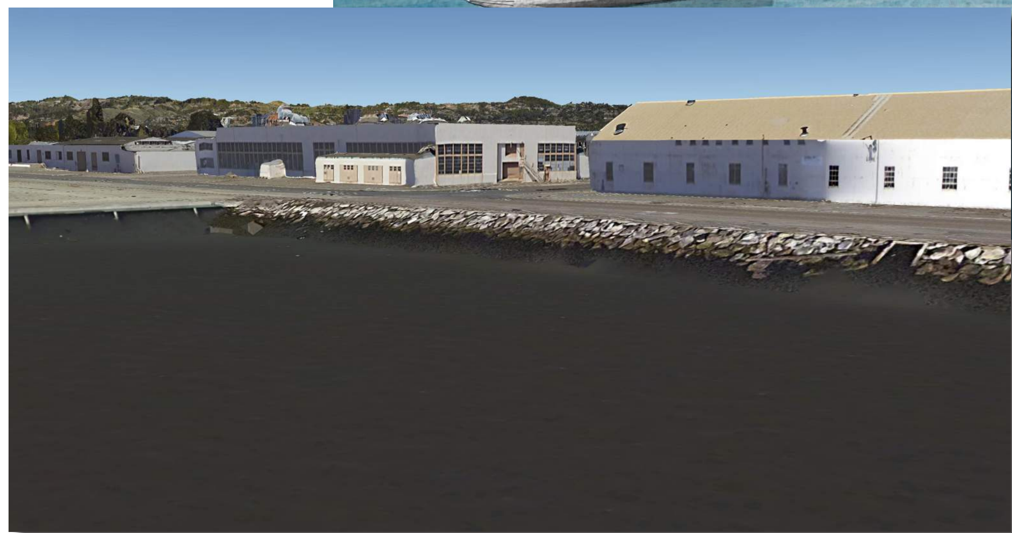
EXISTING CONDITIONS - BUILDING 113
