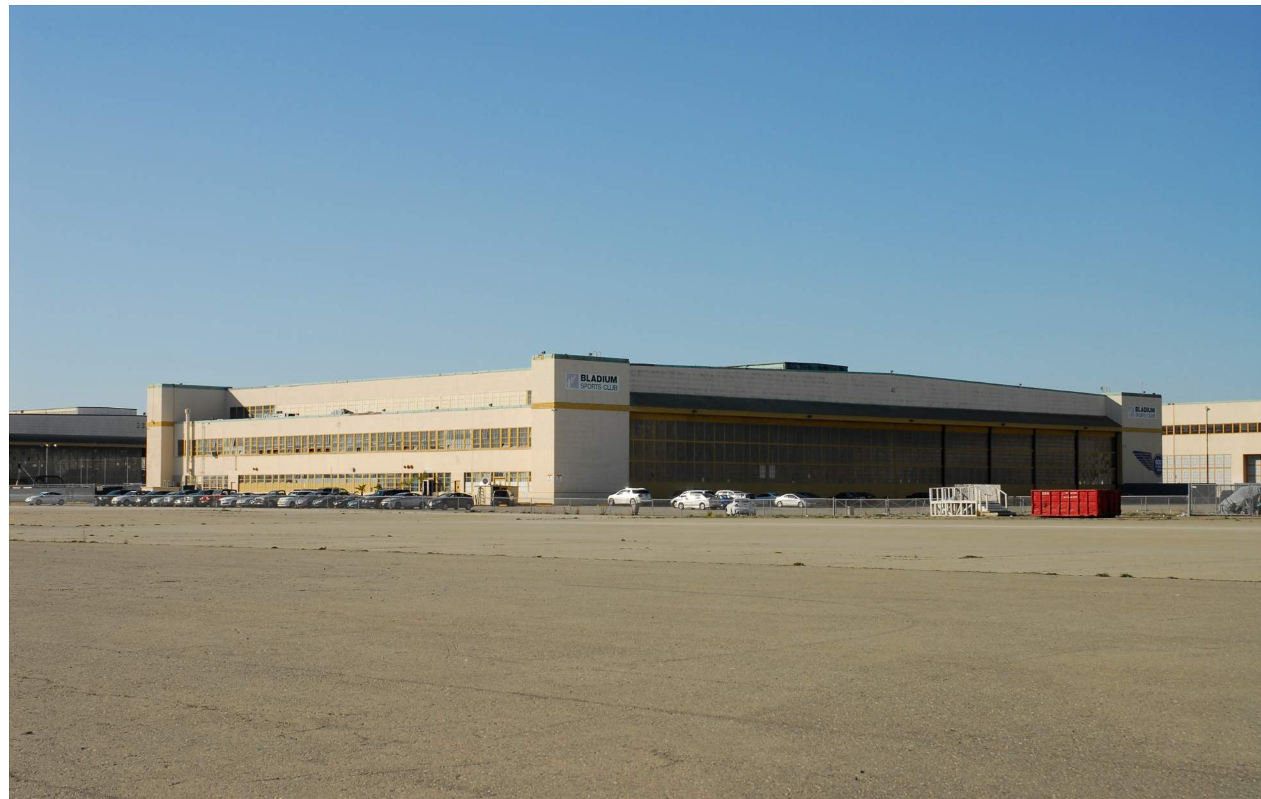
EXISTING BUILDING 40 (BLADIUM)
