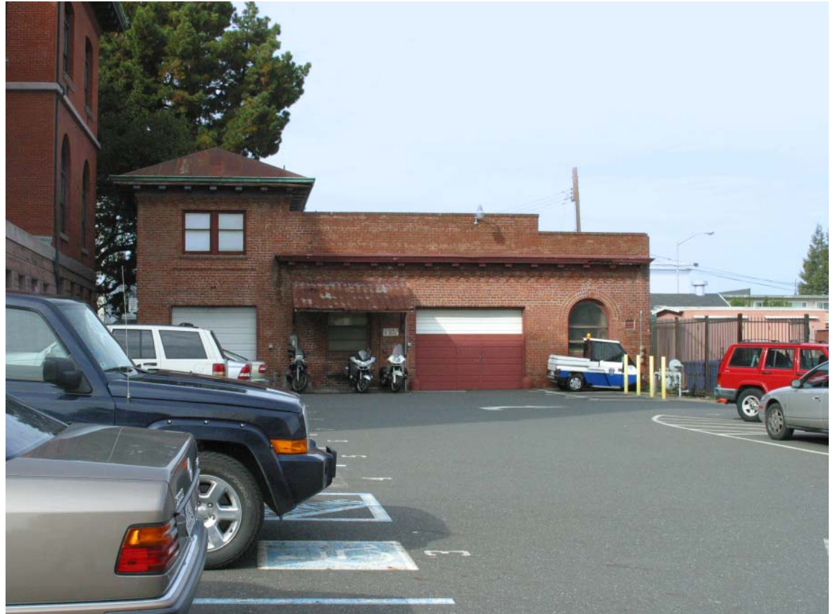
ABOVE Existing parking lot
