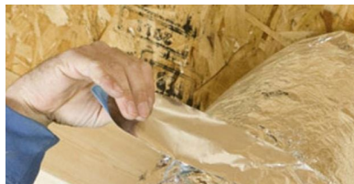
Duct Sealing, New Ducts, and Duct Insulation
