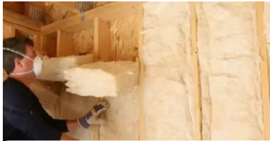
Wall, Attic, and Rase Floor Insulation
