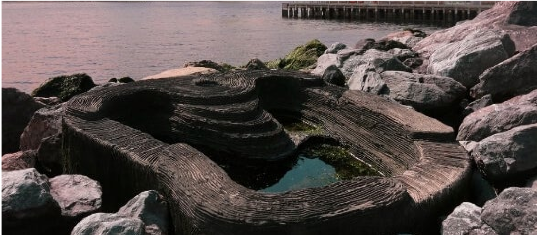
E-concrete textured armoring
