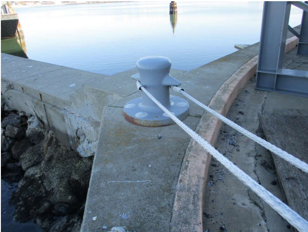
Photo 6 - Typical condition new mooring bollard at Pier 1
