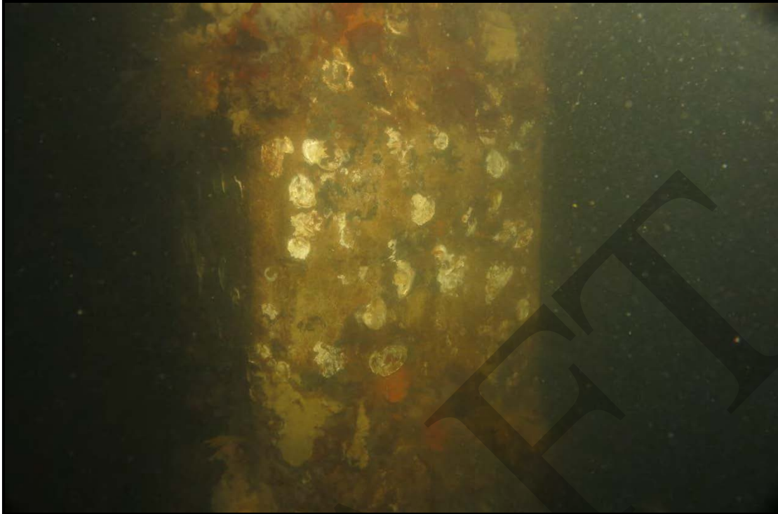
Photo 5: Typical Level II location with marine growth removed.
