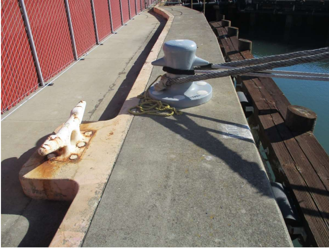
Photo 7 - Typical condition curb and new mooring bollard at Pier 1
