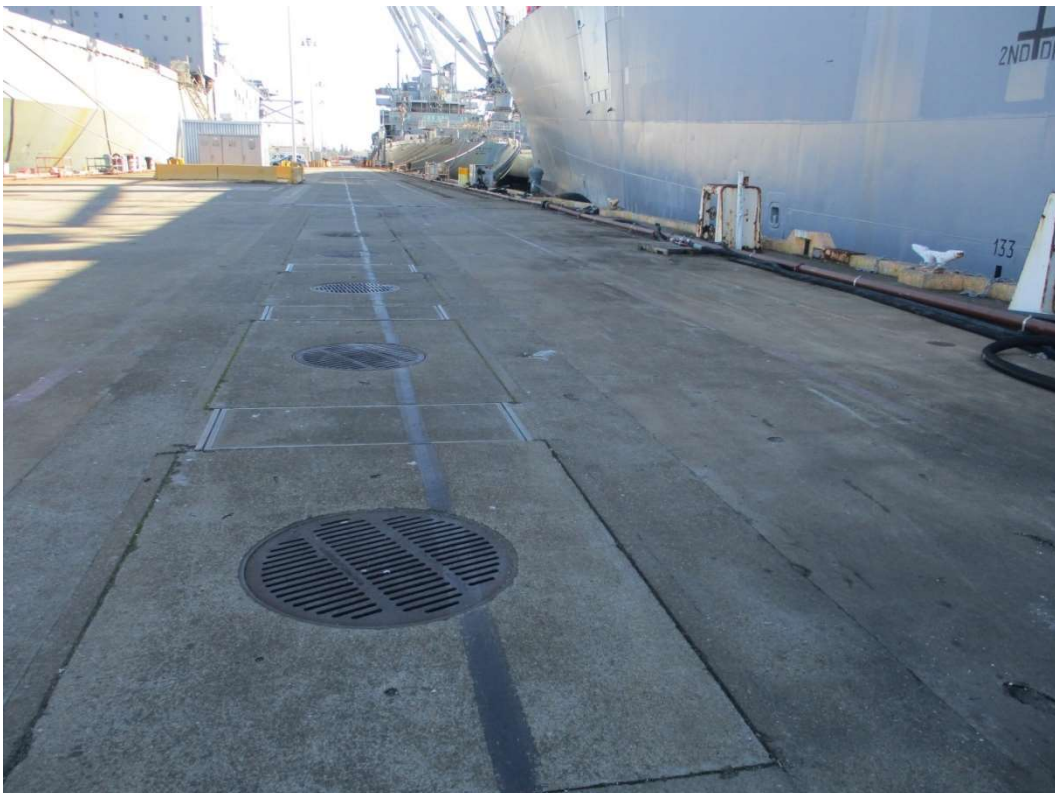
Photo 14 - Typical condition of deck at Pier 2
