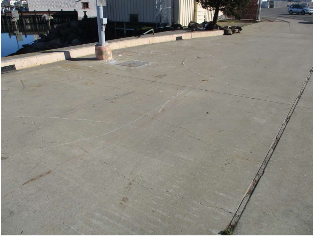
Photo 3 - Typical condition of deck at Pier 1
