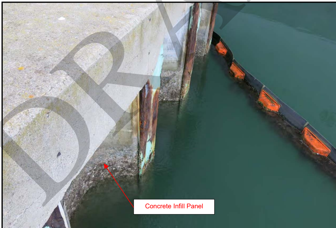
Photo 2: Scalloped concrete infill panels at south side of Pier 1.
