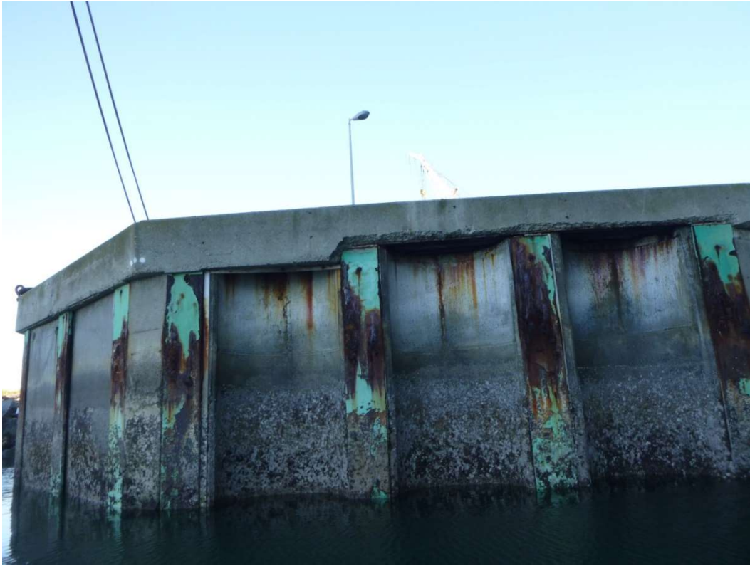
Photo 1 - Typical above water condition of king piles at Pier 1
