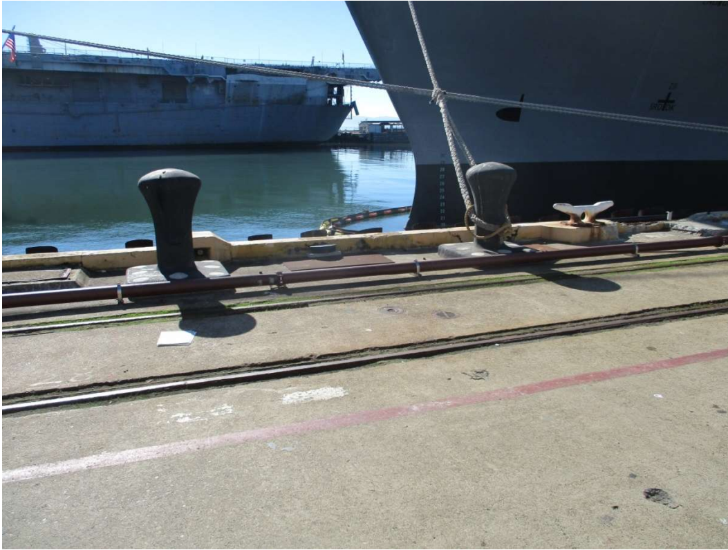
Photo 19 – New bollards at Pier 2
