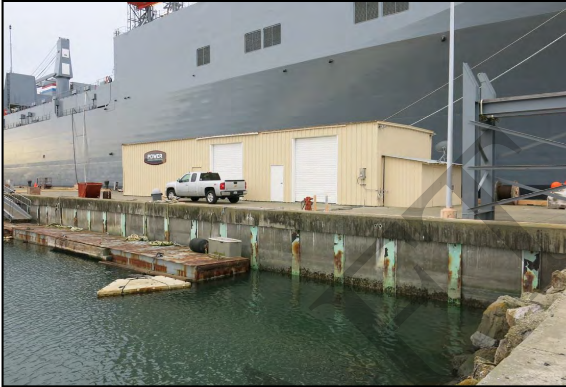
Photo 3: Flat concrete infill panels at north side of Pier 1.
