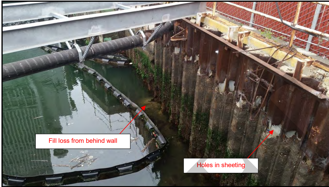
Photo 7: Original steel sheet pile wall at south side of Pier 1.
