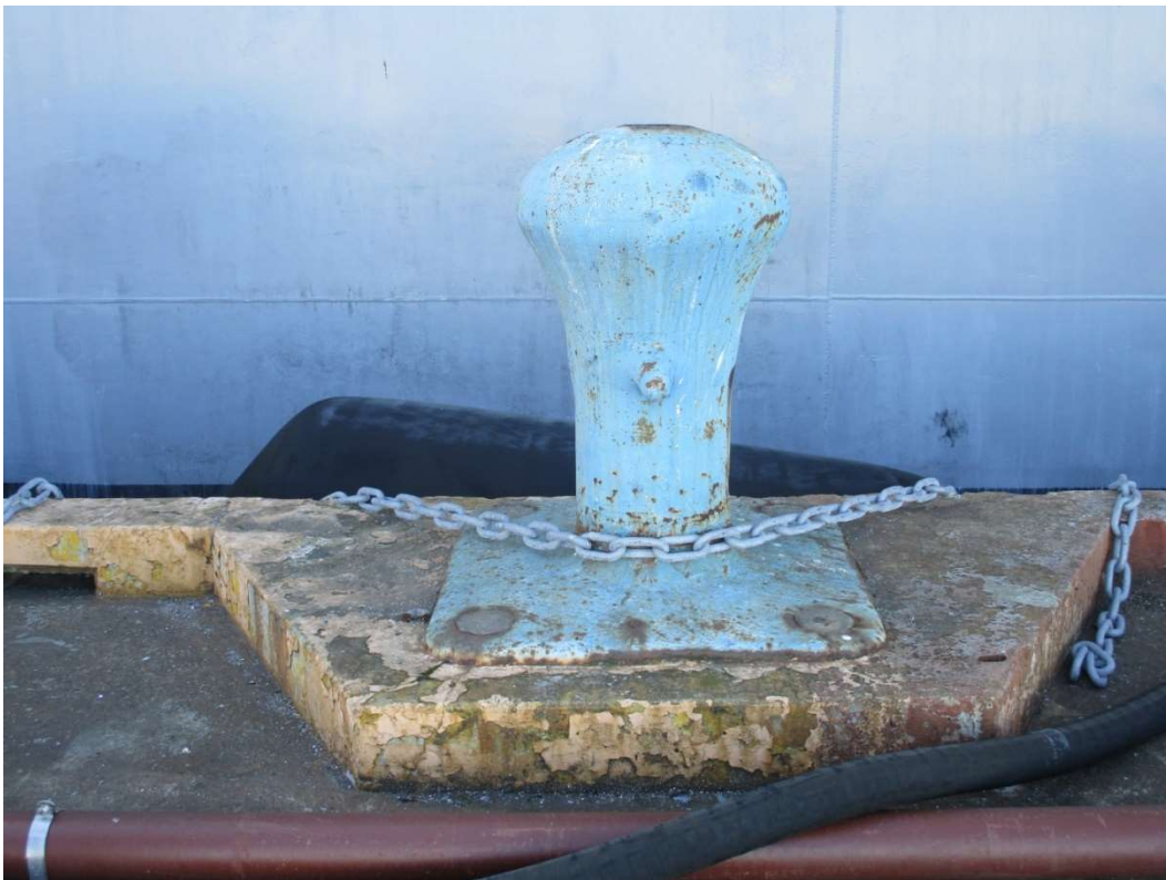
Photo 16 - Typical condition of mooring bollard and base at Pier 2
