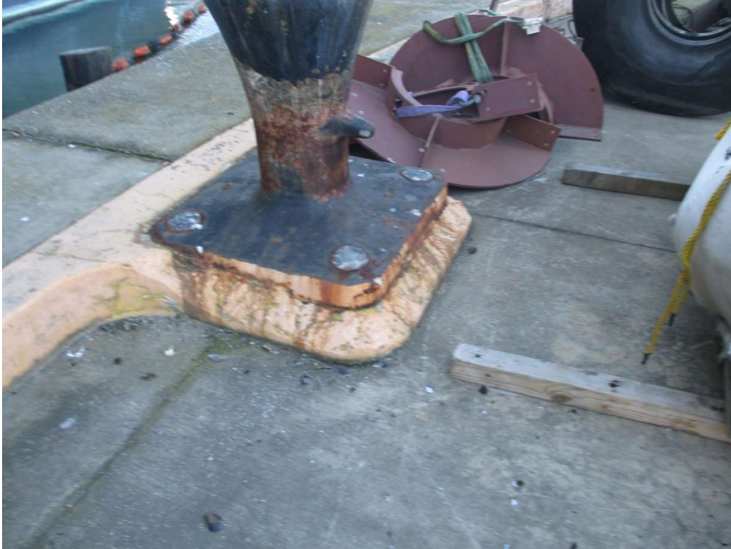
Photo 5 - Typical condition of mooring bollard and base at Pier 1
