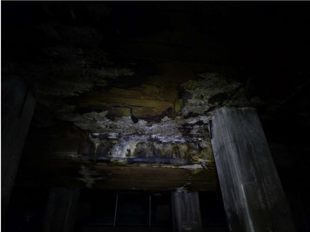
Photo 23 – Efflorescence at soffit of Pier 3
