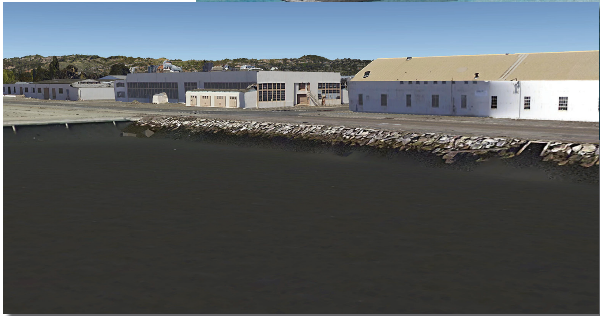
EXISTING CONDITIONS - BUILDING 113
