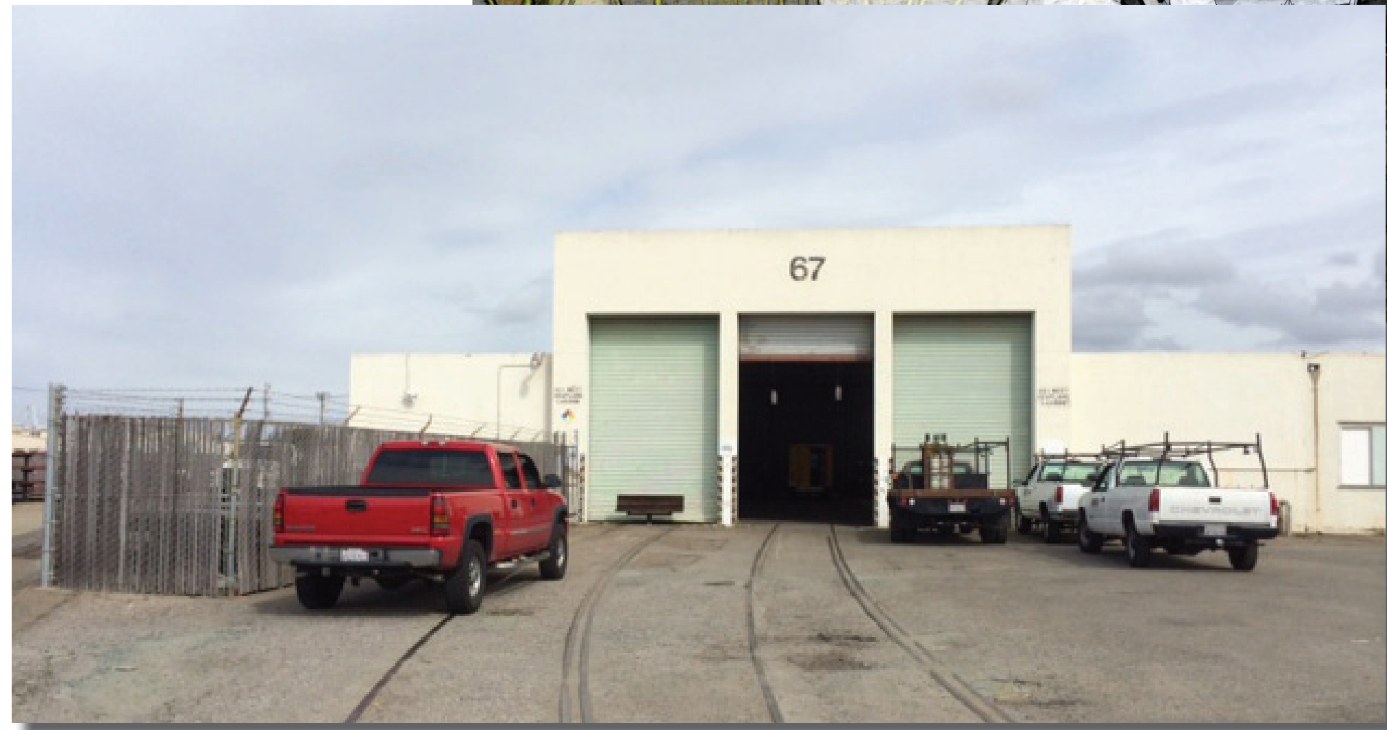
EXISTING CONDITIONS - BUILDING 67
