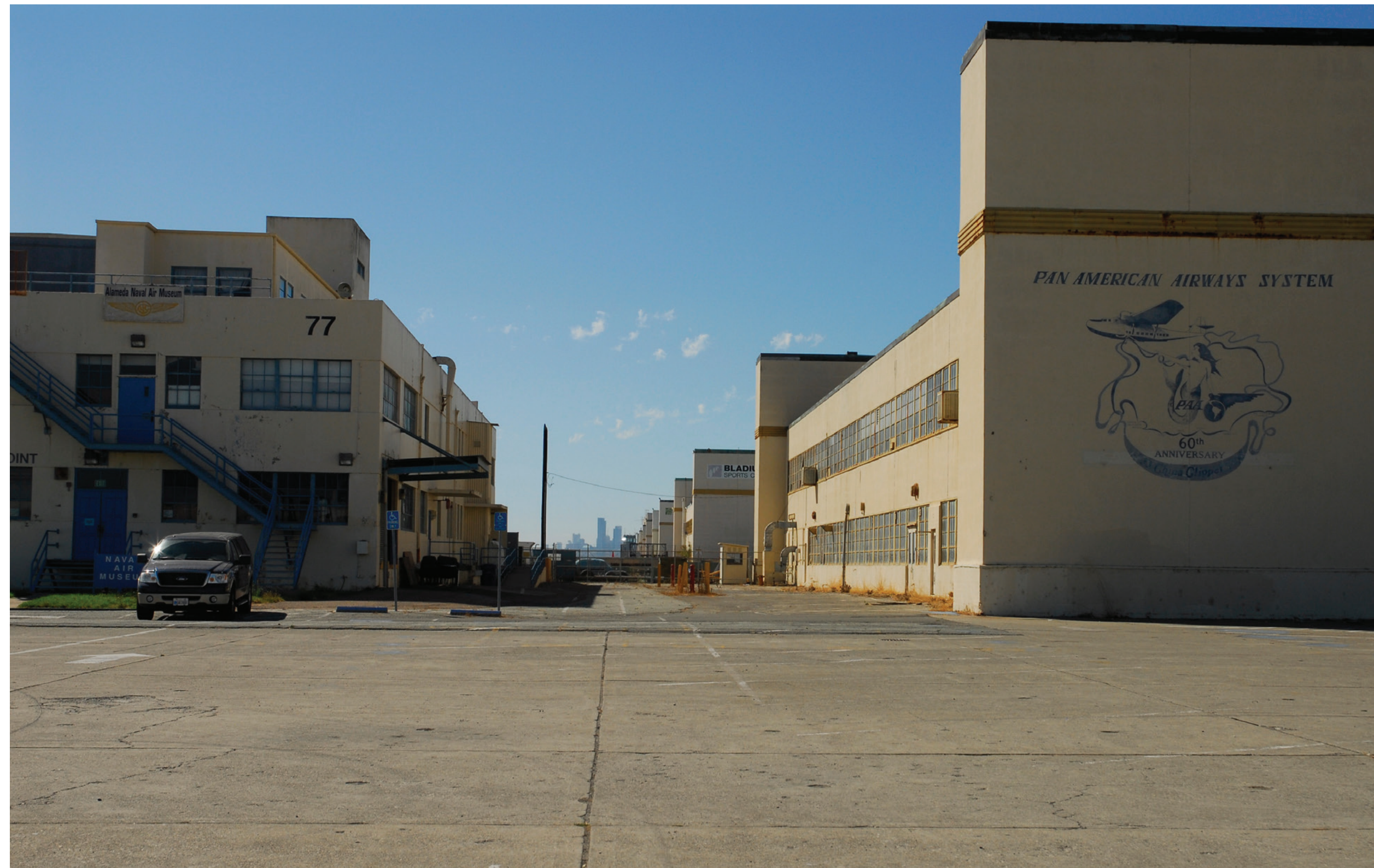
EXISTING BUILDING 77 (LEFT) AND 41 (RIGHT)
