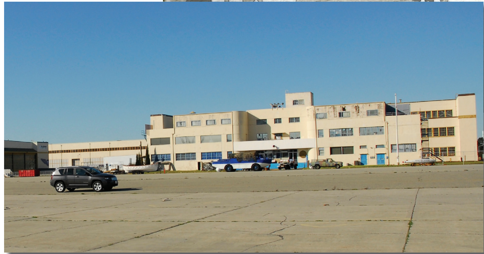
EXISTING CONDITIONS - BUILDING 77
