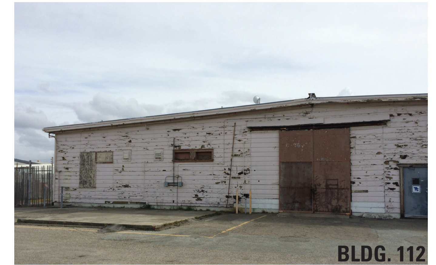
EXISTING BUILDING PHOTOS
