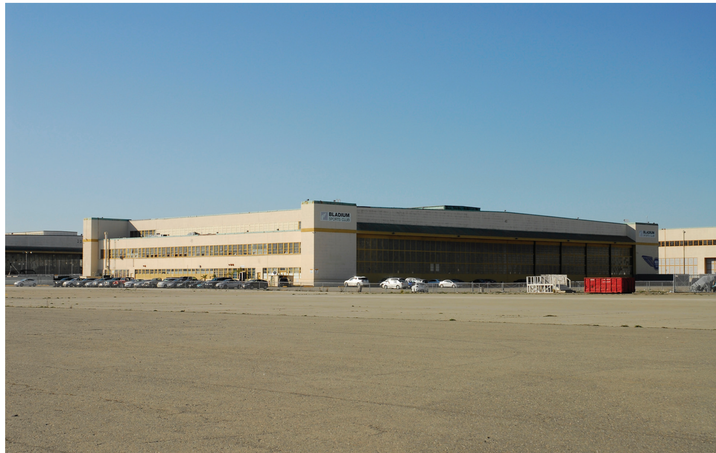
EXISTING BUILDING 40 (BLADIUM)
