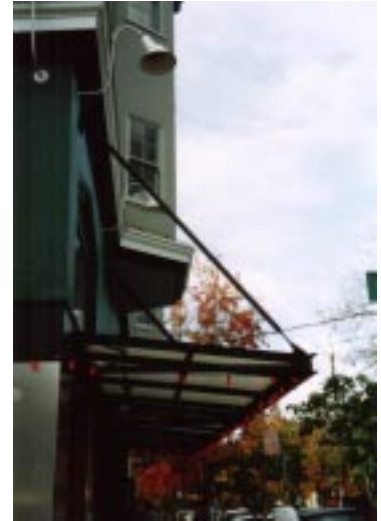
Guideline 8.1: Encouraged - Metal-framed glass awning.
