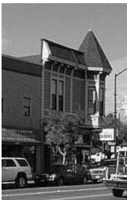
Guidelines 2.3 and 2.4: Pent roof above cornice.
