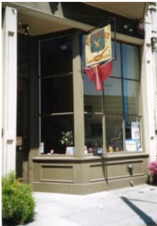
Guideline 6.12: Restored Victorian storefront with wood bulkhead and wood sill.
