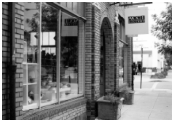
Guideline 6.17: This storefront features pressed brick.
