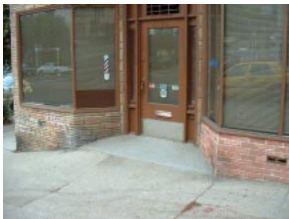
Guideline 6.17: This storefront features pressed brick.
