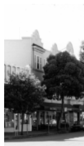
Guideline 2.2: Encouraged - Use parapets to conceal flat roofs.
