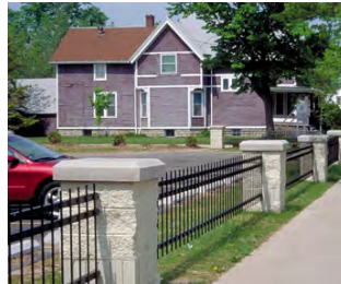
Masonry piers, caps, and ironwork.
