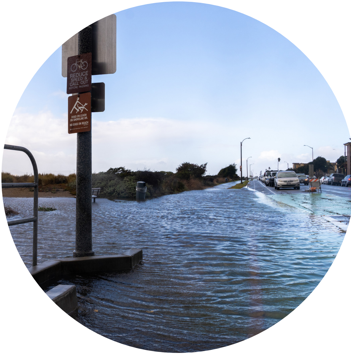
Coastal flooding along the Alameda Beach Bay Trail
