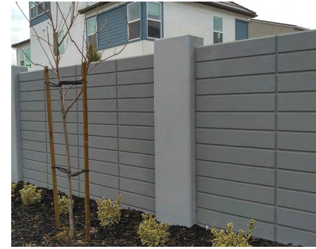
SOUNDWALL AT PROPERTY LINE
