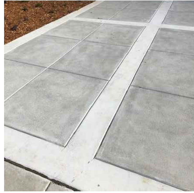
DECORATIVE CONCRETE AT GATHERING SPACE
