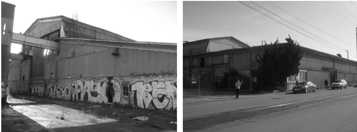
Figure 4.E-2 Steel Fabrication Shop and Warehouse. (left - rear) and (right - front & side)
