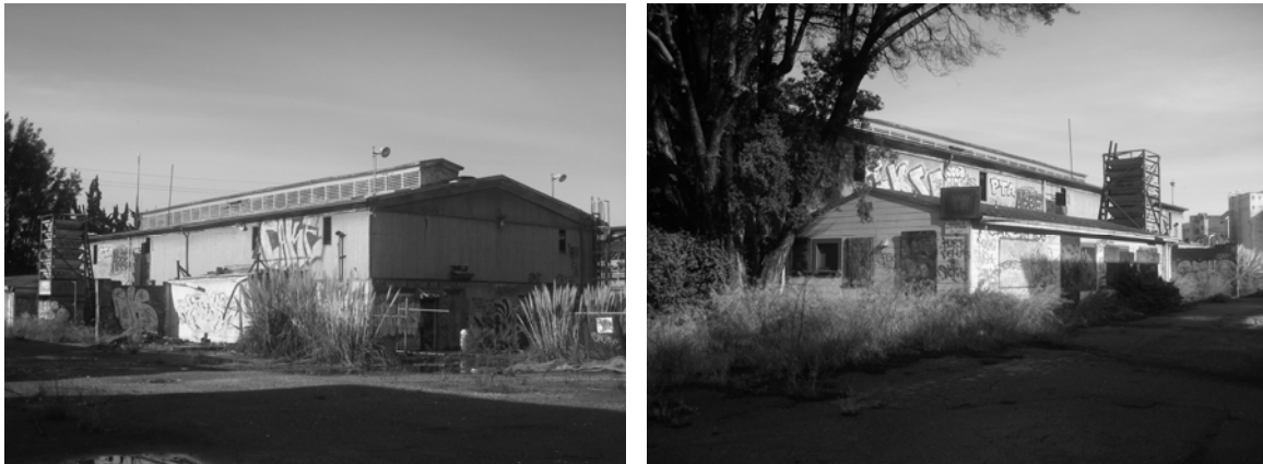
Figure 4.E-4 Compressor Room/Storage Building (left - rear & side) and First Aid Office (right - front & side)
