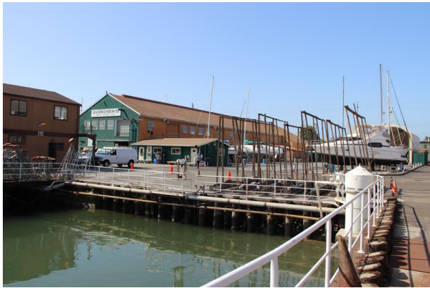
Figure 9. Typical bulkhead wharf at Alameda Marina, 2016.
