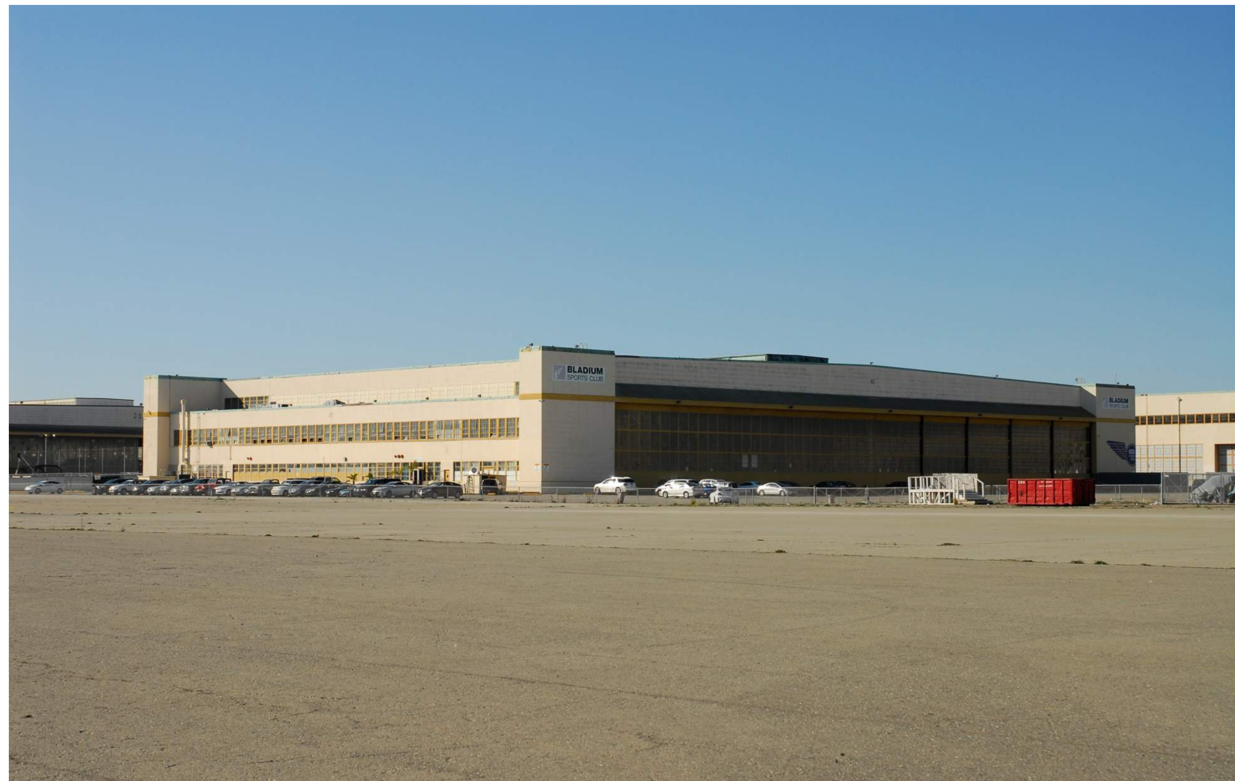
EXISTING BUILDING 40 (BLADIUM)
