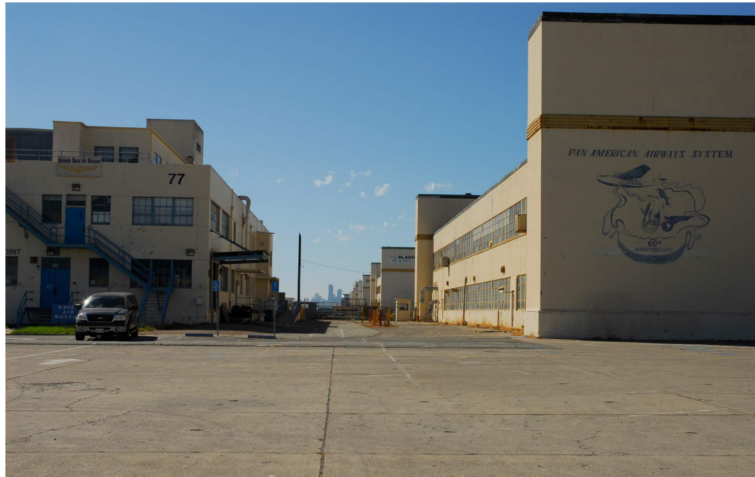
EXISTING BUILDING 77 (LEFT) AND 41 (RIGHT)
