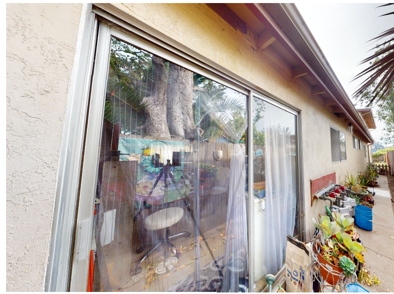
View @ North-West Front Corner
