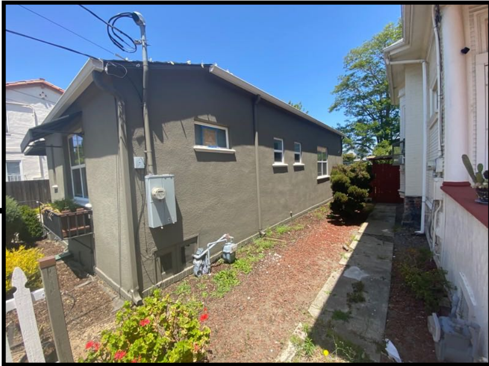
EAST SIDE LOOKING WEST
