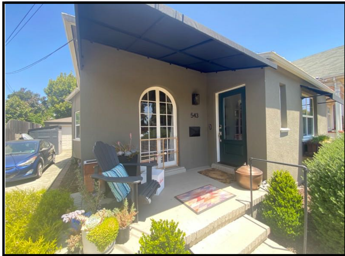
SOUTH WEST FRONT PORCH
