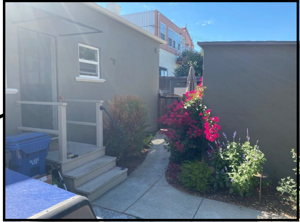
BACK YARD BETWEEN GARAGE & HOUSE LOOKING WEST
