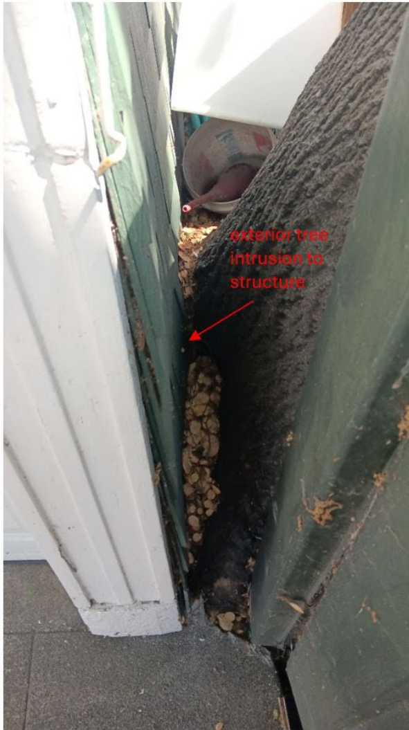
Photo 2. Outside and inside structure view of tree intrusion to garage structure
