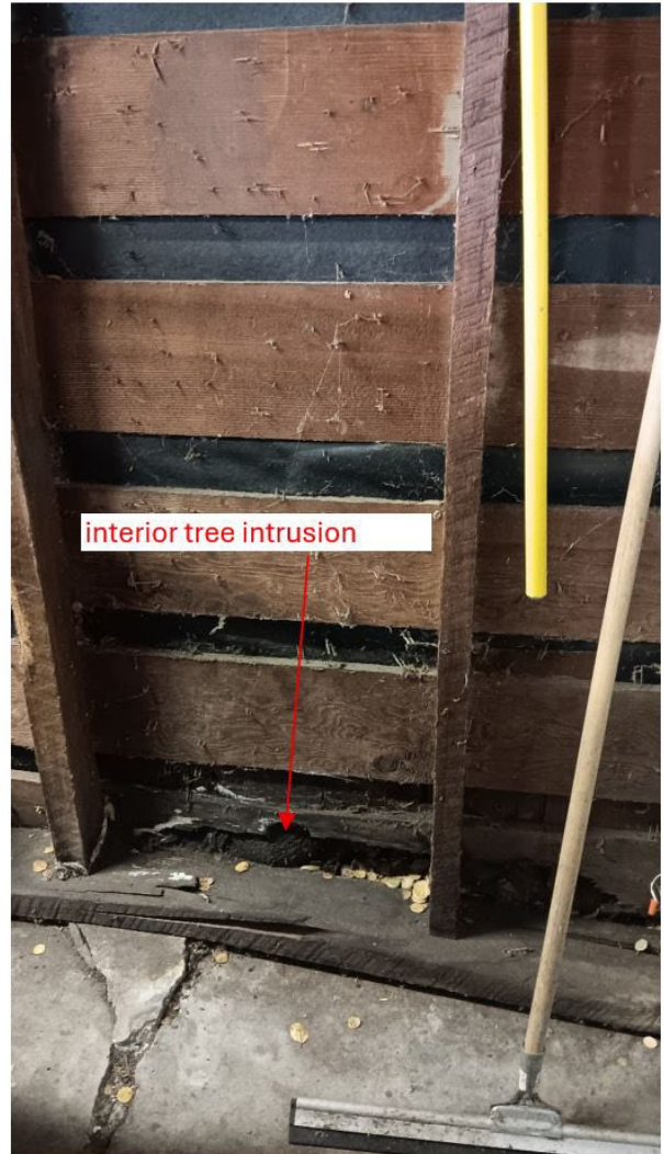
Photo 2. Outside and inside structure view of tree intrusion to garage structure
