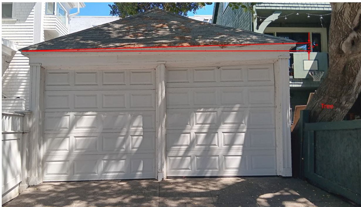
Photo 1. Street view of garage structure, showing tree lean and garage vertical displacement.
