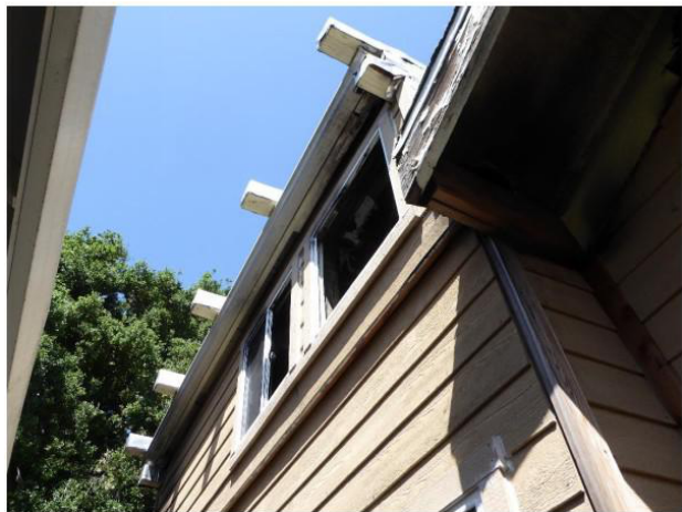
Figure 17: Exposed rafters at upper floor of south façade.
