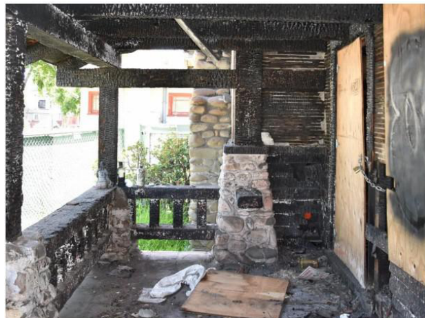
Figure 7: Burn-damaged porch, looking east. Main entry to the house at right.
