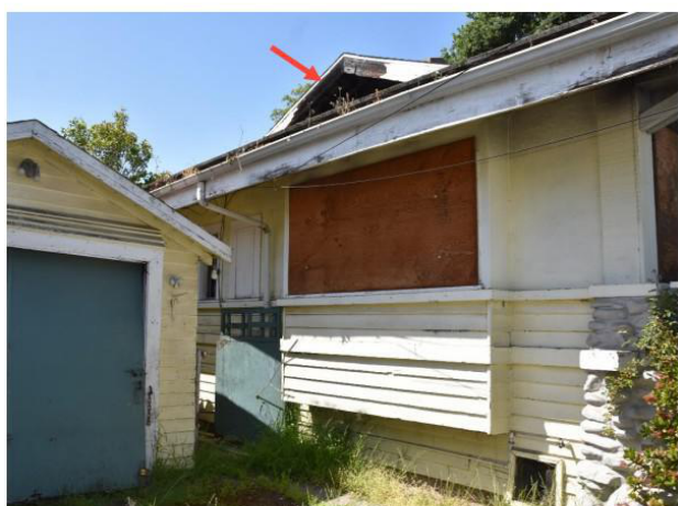
Figure 12: East façade next to driveway. Burn-damaged cross gable above.
