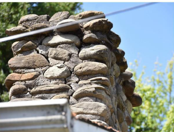
Figure 3: East side of chimney above roofline with cracks and loose mortar.
