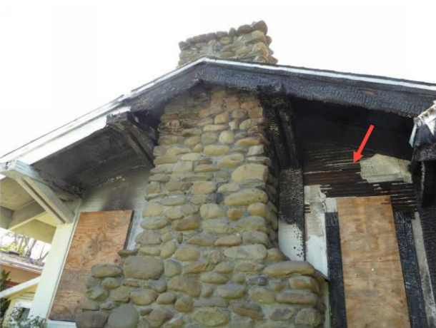
Figure 2: Fieldstone chimney, covered windows, burn-damaged wood elements, and missing stucco.
