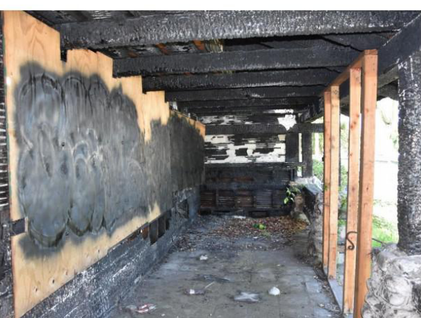
Figure 6: Burn-damaged porch, looking west. Covered window openings at left.
