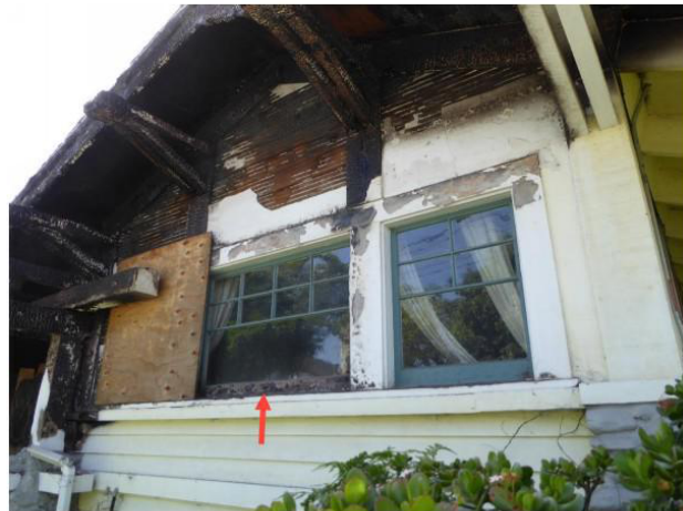
Figure 8: Extant wood windows at west end of north façade. Center window has a burn-damaged bottom rail.
