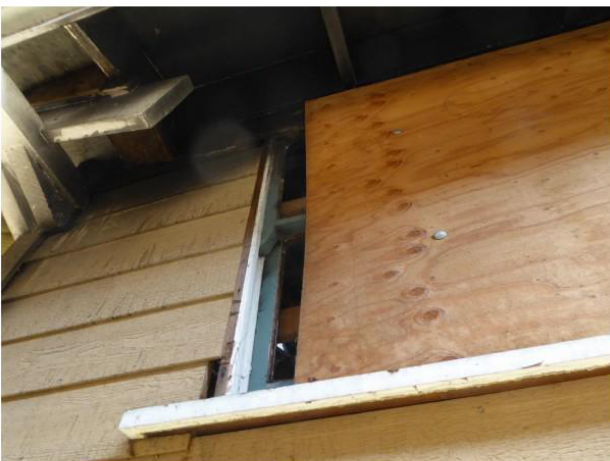
Figure 16: Wood double-hung window behind plywood cover.
