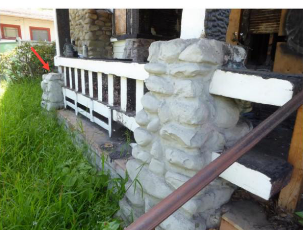
Figure 5: Painted fieldstone porch piers missing stones at furthest east pier.
