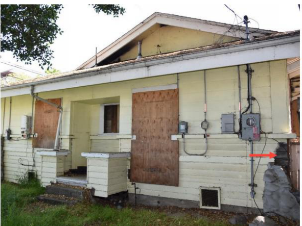
Figure 10: West façade facing Eighth Street. Southwest corner pier with missing stones.
