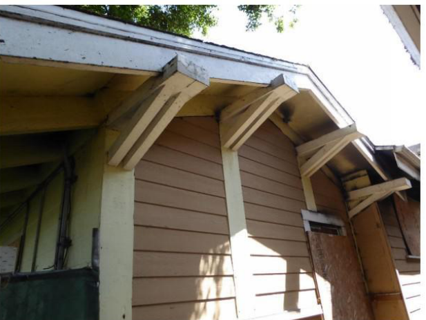
Figure 14: West end of south façade with wood knee braces in good condition.
