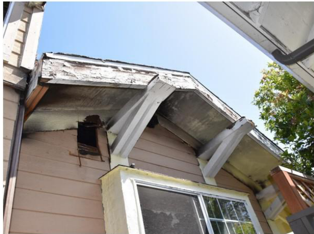
Figure 18: East end of south façade with wood knee braces in fair condition.
