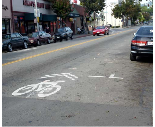
Figure 16. Use of parking T's along Class II and Class III bikeways to help bicyclists identify and steer clear of the “door zone” of parked vehicles. (source for diagram: City of Oakland)
