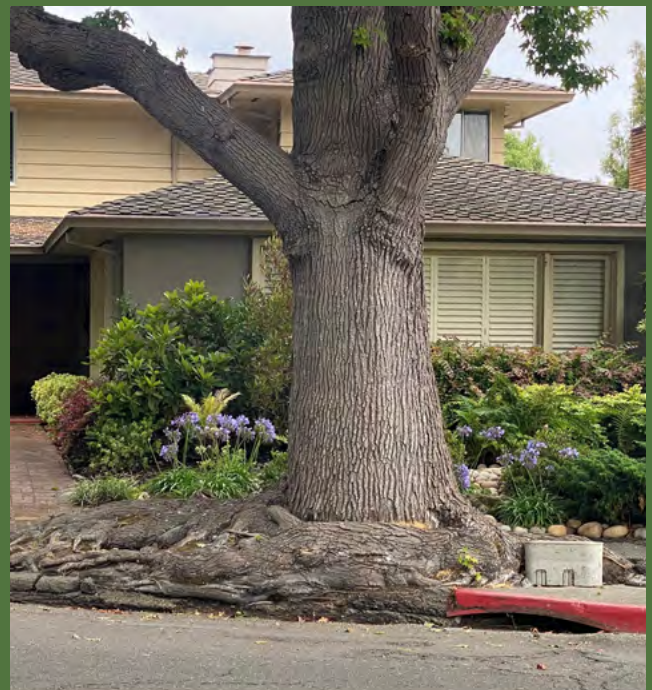
Photo 4: Roots from tree #1539 damaged hardscape on all sides of the trunk. Note pillowing over curb and sidewalk.
