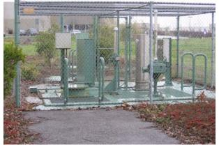
**Existing Equipment:** System I: Unknown System II: Prime Pump No. 20P16A-11.5, 60 hp, 1170 RPM
