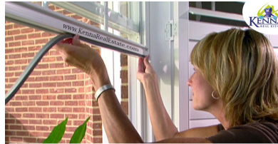
Air Sealing and Weather-Stripping
