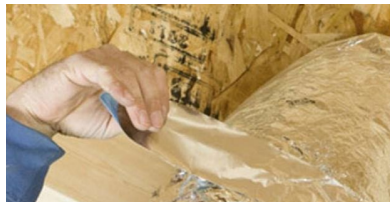
Duct Sealing, New Ducts, and Duct Insulation
