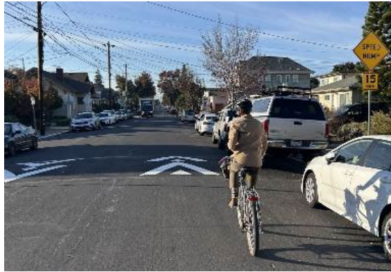
Asphalt Speed Hump
