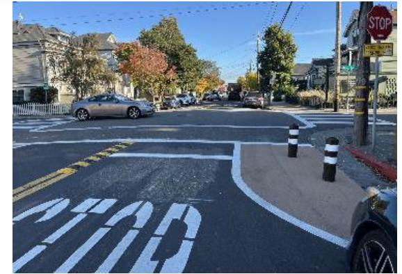
Painted Bulb-out with Hardened Centerline
