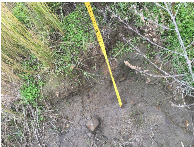
Figure 4 - Minor erosion on side slope
