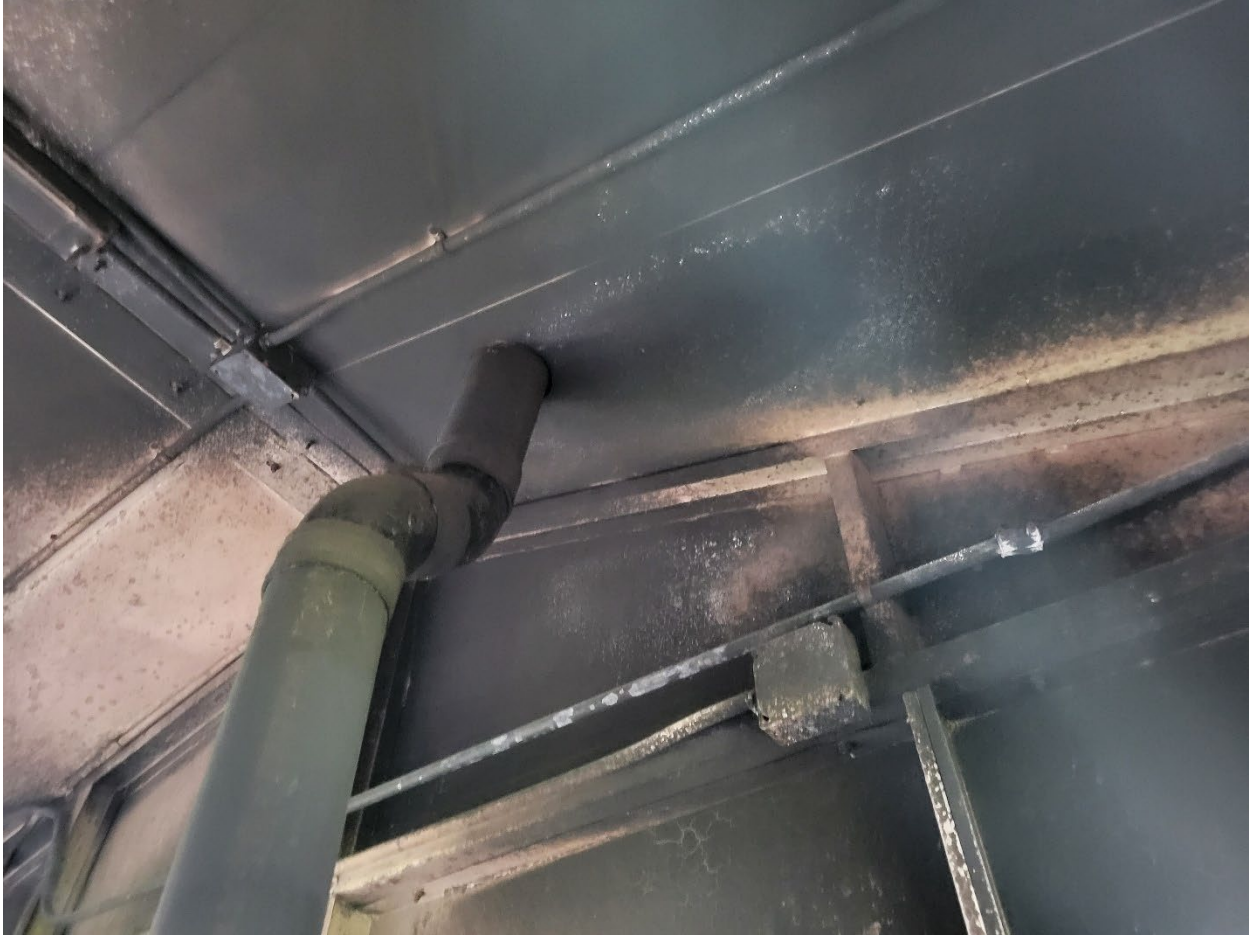
Figure 6 Harrington Utility Closet Ceiling 1
