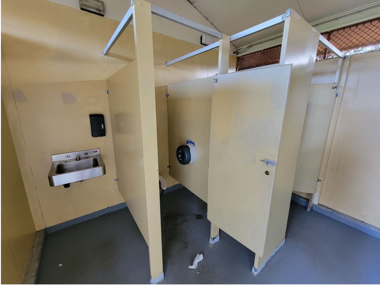
Figure 28 Harrington Women's Restroom General View
