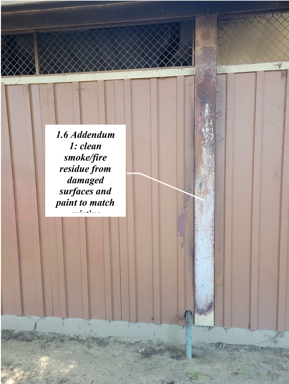
Figure 24 Addendum 1: Exterior Cleaning and Paint repair – rear wall
