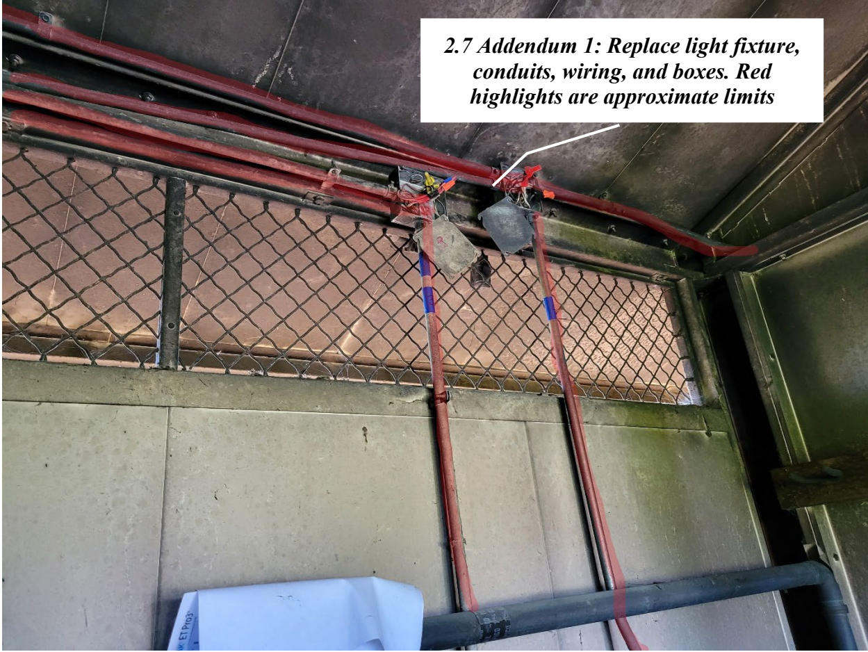
Figure 12 Addendum 1:Harrington Utility Closet Electrical
