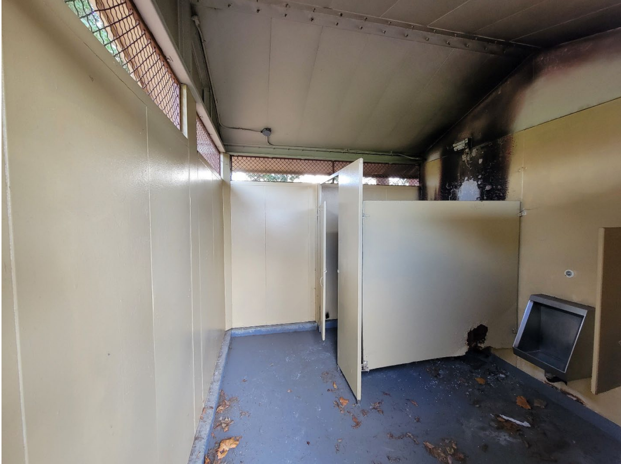
Figure 13 Harrington Men's Restroom Interior General View
