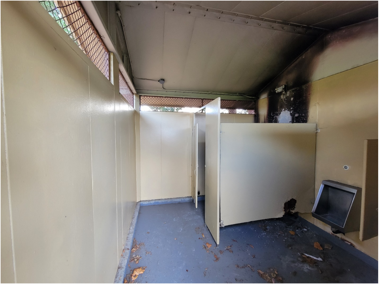
Figure 10 Harrington Men's Restroom Interior General View
