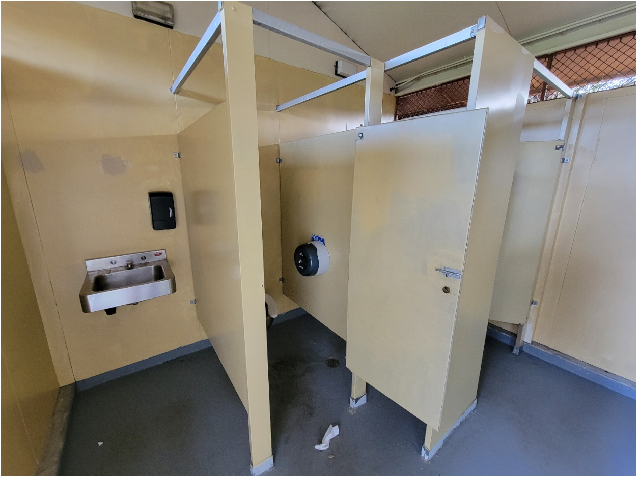
Figure 21 Harrington Women's Restroom General View
