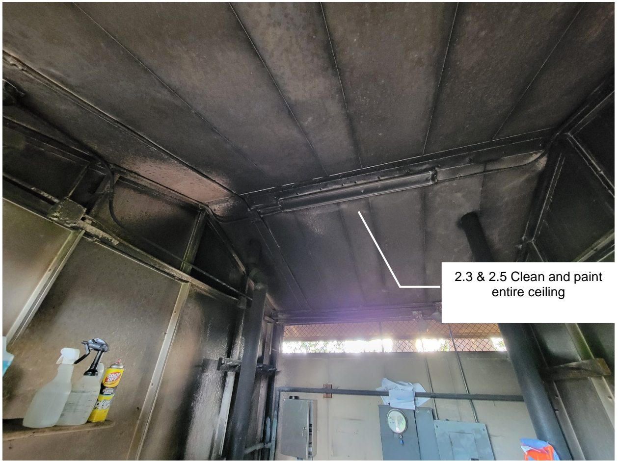
Figure 5 Harrington Utility Closet Ceiling 2
