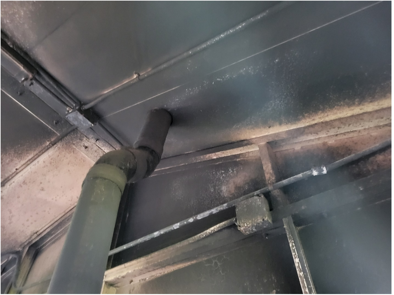
Figure 6 Harrington Utility Closet Ceiling 1
