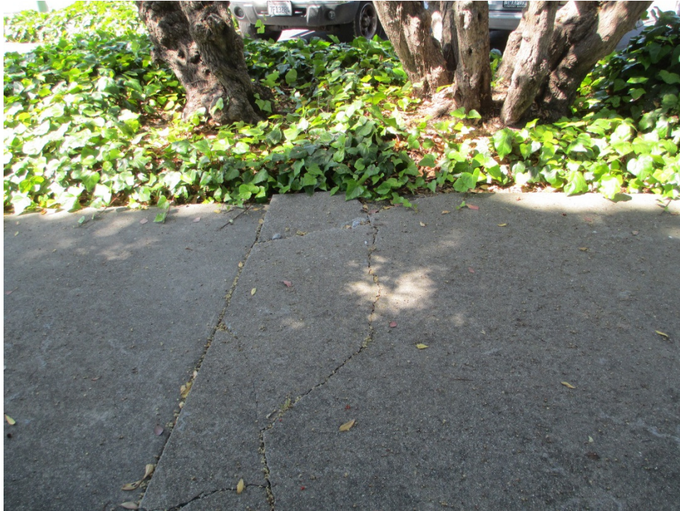
Photo 4. Photo to the left shows the bases of Myoporum trees #8 and 9, and the adjacent root related hardscape displacement. The trees are infested with Myoporum Thrip . The trees are expected to decline at an increasing rate if root loss occurs.
