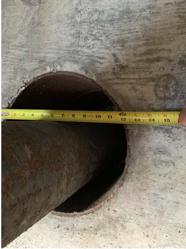
Photos 1 & 2: Cola Ballena Bridge Abutment Penetration (south side)
