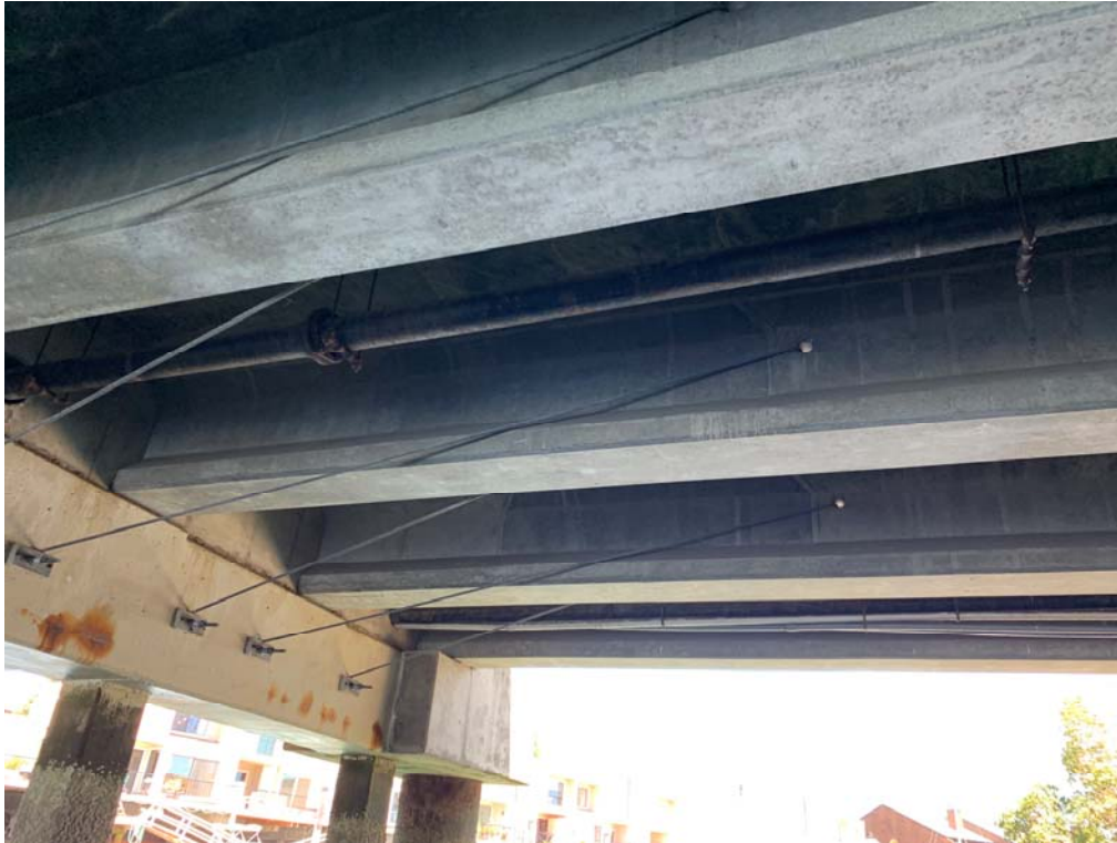
Photo 4: Cola Ballena Bridge – Force Main Under Bridge
