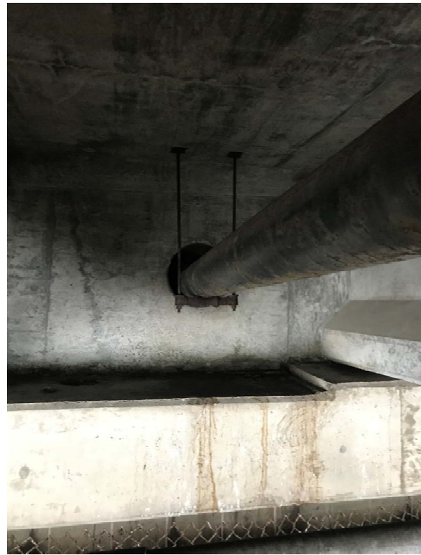
Photos 1 & 2: Cola Ballena Bridge Abutment Penetration (south side)
