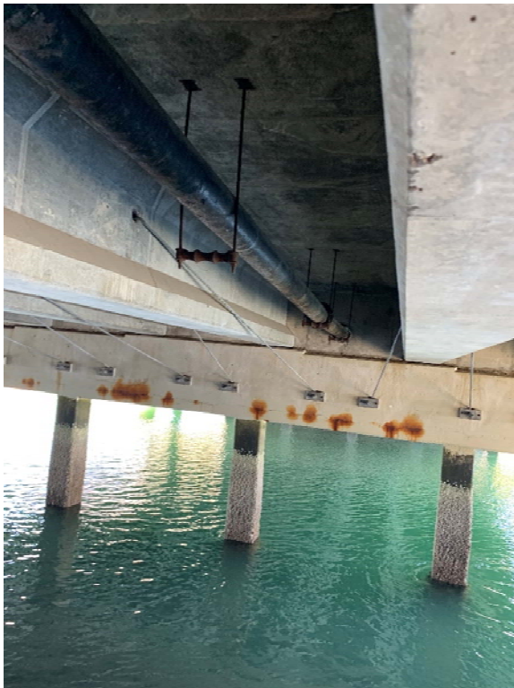
Photo 3: Cola Ballena Bridge – Force Main Under Bridge
